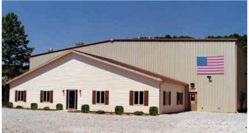
For over 20 years Hydraulic Specialists Inc. of Midvale, OH has offered quality workmanship, competitive pricing and fast turn around on repair of hydraulic cylinders, pumps, and motors.
